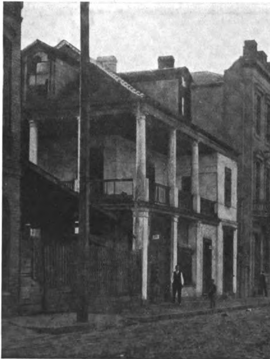
OLD HOUSE NEAR LEE CIRCLE
