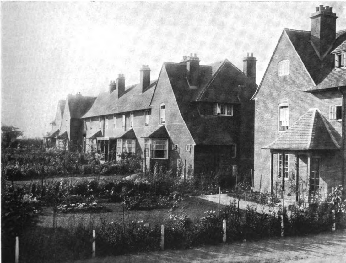
REAR YARDS—HAMPSTEAD GARDEN SUBURB
