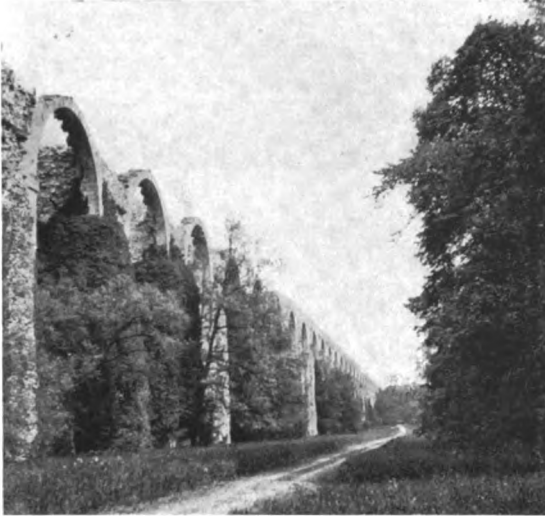
THE AQUEDUCT OF MAINTENON
