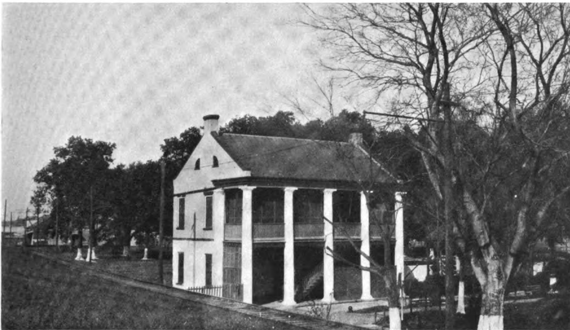
OFFICERS' QUARTERS, JACKSON BARRACKS, NEW ORLEANS, WHICH WOULD BE TOTALLY DEMOLISHED TO MAKE WAY FOR THE NEW ROADWAY. See page 129
