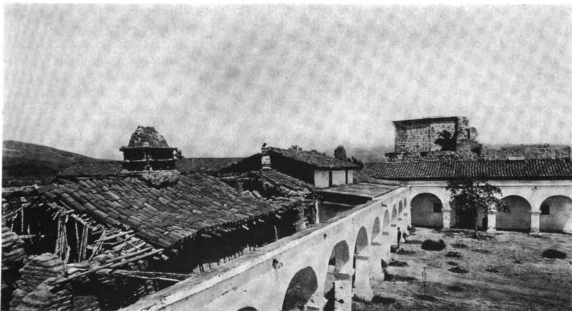
KITCHEN CHIMNEY AND ROOF.—SAN JUAN CAPISTRANO
