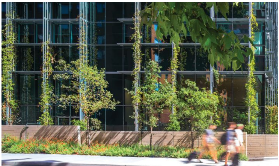
The Edith Green-Wendell Wyatt Federal Building in Portland, Ore., by SERA Architects and Cutler Anderson Architects is a 2014 COTE Top Ten winner that serves as an example of a high-performing renovation and retrofit.
