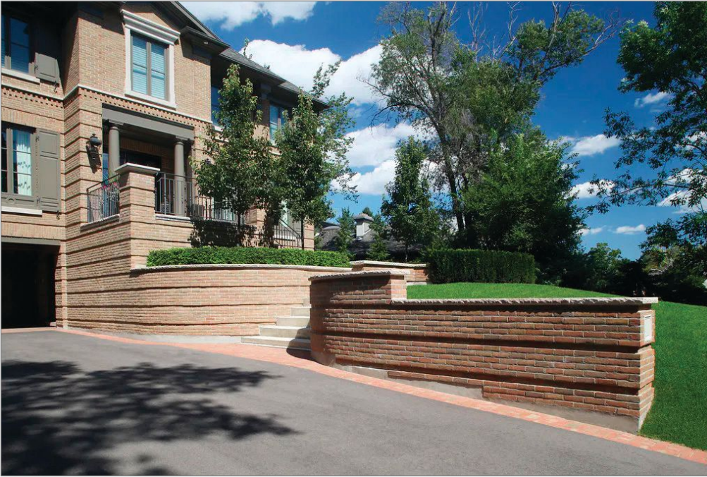
Angling brick to achieve a radius only works in stack bond construction; if a running bond is used, the edges of the brick units in one course will project over brick faces in adjacent courses.
