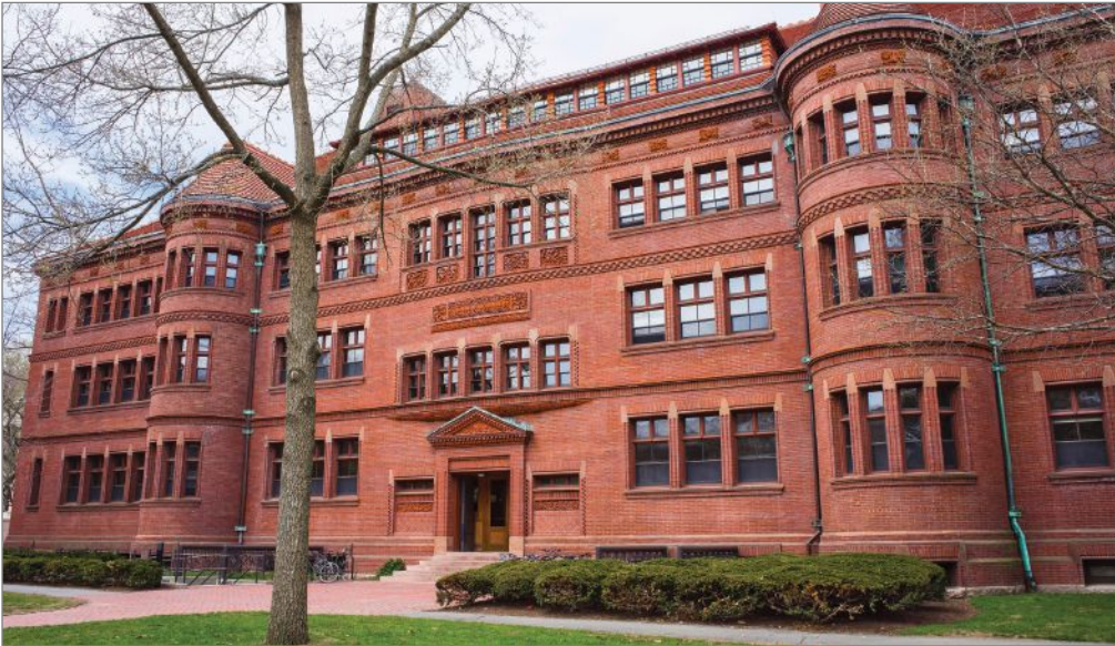
The Romanesque Revival style of architecture, which was popular from approximately 1870 to 1900, employed massive brick arches over windows and entryways, round brick turrets, load-bearing masonry walls, corbelling, and multicolored facades created with contrasting building materials such as brick and stone or several different colors of brick.
