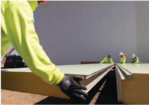
Insulated roof deck panels can achieve R-values ranging from 16 to 62, depending on the product thickness, which ranges from 2 to 8 inches.
