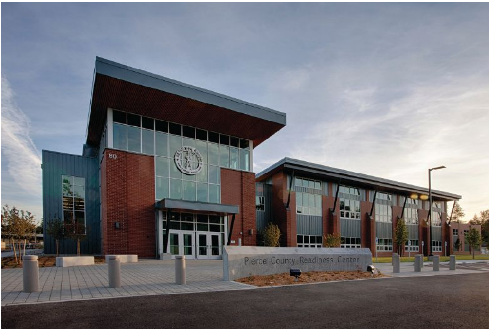
Pierce County Readiness Center. Photo: WJA Design Collaborative / Ric Peterson Photography
