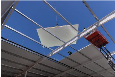
Insulated roof deck systems save time and labor costs, are more energy efficient, and—when paired with a patented mechanical panelizer system—improve job site safety compared with traditional low-slope roofing products.
