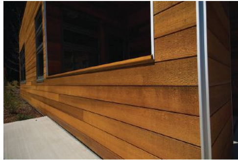
The different joints and surface textures in tongue and groove siding combine to provide a range of shadow line effects that enhance the product's versatility; the image on the left shows a flush joint tongue and groove, while the image on the right is a fineline tongue and groove.
