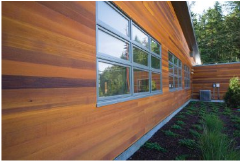
The different joints and surface textures in tongue and groove siding combine to provide a range of shadow line effects that enhance the product's versatility; the image on the left shows a flush joint tongue and groove, while the image on the right is a fineline tongue and groove.
