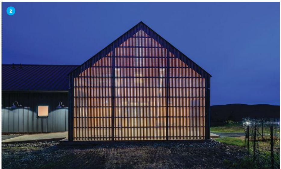
1. The podium of the bank barn-inspired cidery is clad in locally sourced bluestone. 2. On the side entry, light filters through larch slats and a protective polycarbonate layer.
