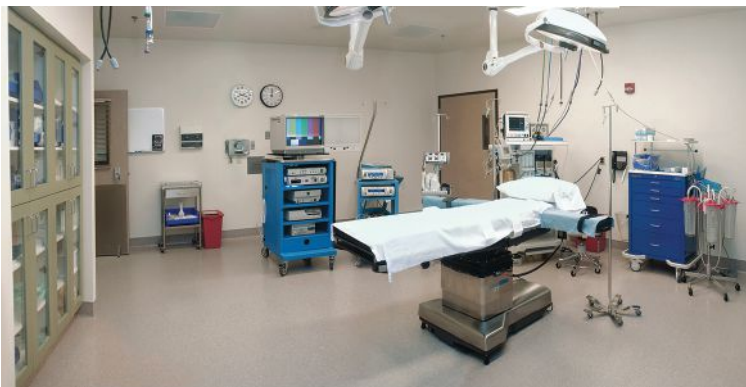
The repeated process of wiping the wall surface with a fibrous disposable material along with the strong concentration of bleach can cause a traditional wall paint to break down and wear away over time.
