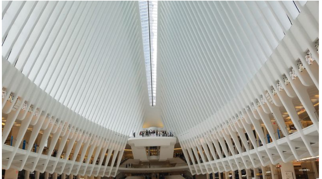
Architecturally exposed structural steel commonly uses intumescent coatings as a method of fire protection. The World Trade Center Transportation Hub (The Oculus) achieved prescriptive design requirements with the use of intumescent coatings. Photo Courtesy of AISC
