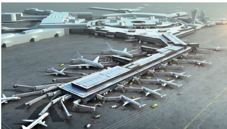
Figure 3. The design team for the San Francisco International Airport expansion used Life Cycle Assessment (LCA) to quantify and reduce environmental impacts. They used product-specific EPDs to demonstrate that the low-cement concrete mixes had significantly lower impact than baseline mixes from the region. As a result, the project earned 3 points for meeting the LEED v4 LCA credit. Architect: HKS; LCA consultant: Arup; Structural Engineer: Rutherford & Chekene; Image: Courtesy of HKS.
