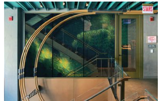
Each floor of this stairwell tells a story about coffee-growing, which is on full display thanks to the floor-to-ceiling expanses and butt-glazing capabilities of 120 minute low iron glass with superior clarity.
