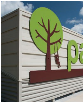
PAC-CLAD REVEAL + HWP METAL WALL PANEL SYSTEMS Color: Sandstone + Granite
