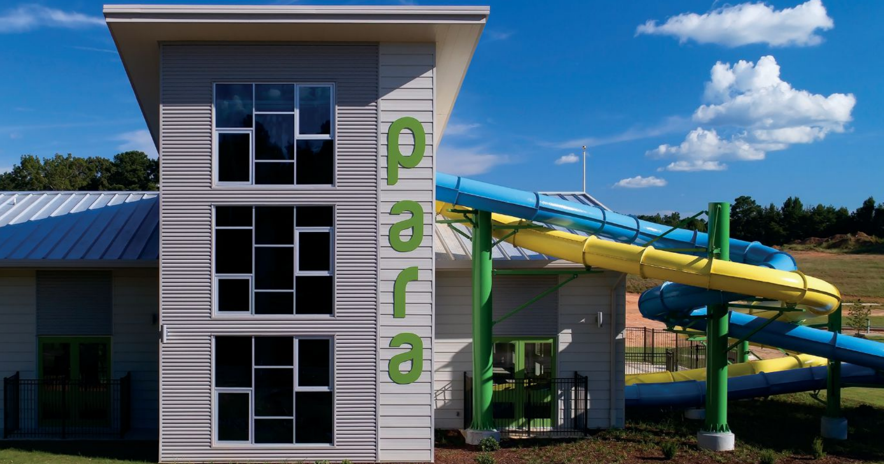
PARA Activity Center, McCalla, AL Installing Contractor: R. B. Atkins & Associates Architect: Ellis Architects Distributor: Roofers Mart Photographer: hortonphotoinc.com Profiles: Reveal panels w/ 2 pencil ribs, HWP panels Colors: Sandstone, Granite
