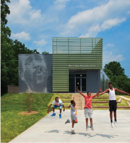
There are three key considerations when creating a fire protection plan: life safety, fire suppression, and protection of the structure. (Pictured the Marvin Gaye Recreation Center) Photo Courtesy of Hoachlander Davis Photography
