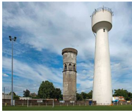
Le Corbusier's Château d'Eau water tower (at center) was erected in the French provincial town of Podensac in 1917 and abandoned in 1940.
