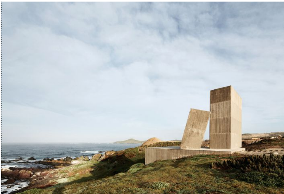
From the south, Casa OchoQuebradas appears as three monumental concrete forms in the landscape.
