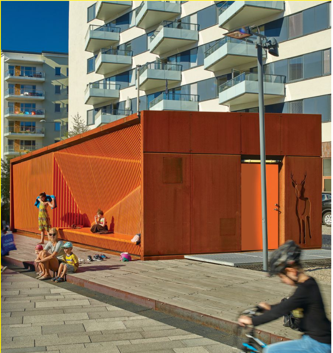
Bottom: The Technical Building, designed by U.D. Urban Design and Anders Ohlin, which houses both an electrical substation as well as pumps for a fountain in Norra Djurgården
