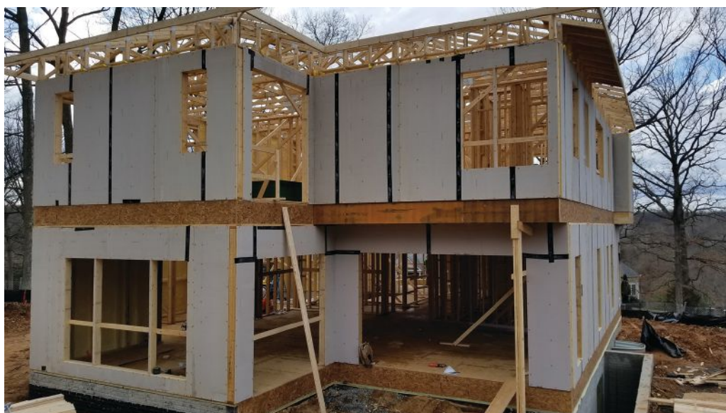
One manufacturer has developed technology to create a wall panel that has more components such as insulation and weather barrier incorporated into a structural wall panel that is built offsite.
