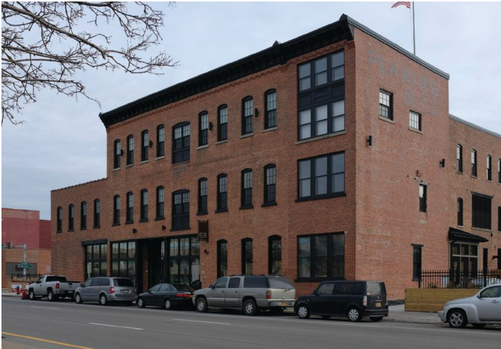
Planning Mill, Buffalo, New York—Adaptive reuse project consisting of loft apartments and retail space. The building was originally built in 1878 and is found in the Registry of National Historic Places.
