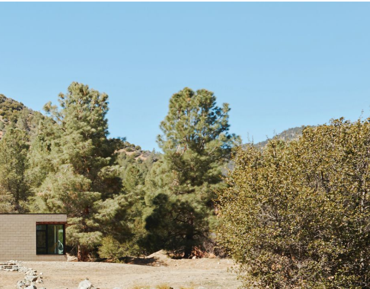
A single-family house in the Mojave Desert is located miles from the nearest utility hookup.
