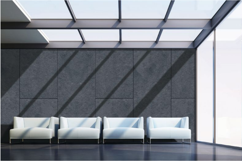
Thin porcelain tile panels are often used in lobbies and corridors, which see a great deal of traffic, for clean aesthetics and durability with fewer grout joints.
