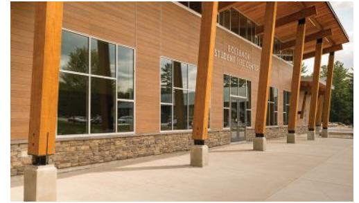
Commercial architectural wall panels (AWPs) are designed and intended exclusively for low- to mid-rise buildings.
