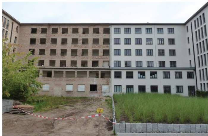
Work underway and completed at Prora
