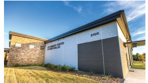
Extruded aluminum adds durability and longevity to construction that other trim materials such as galvanized steel and polyvinyl chloride (PVC) lack. Photo courtesy of Nichiha
