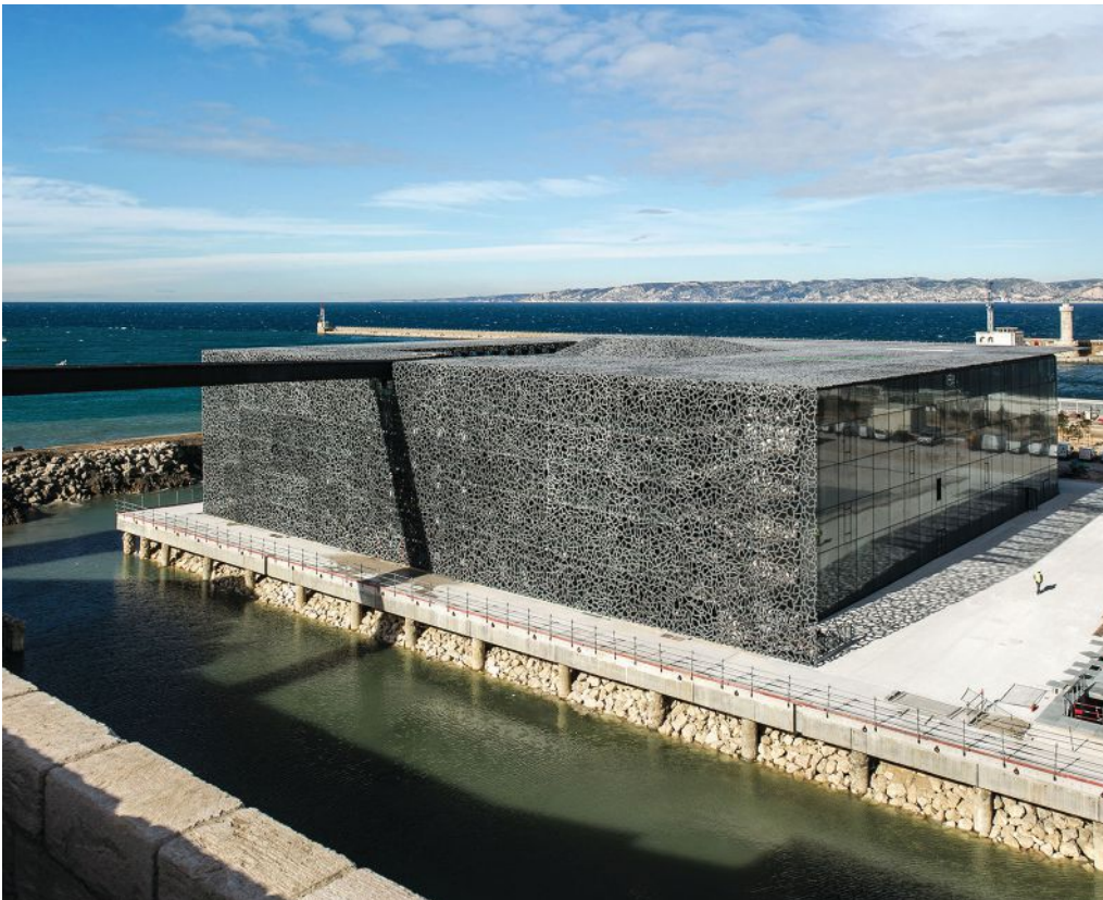
Figure 1: MuCEM, Marseille, France. A unique UHPC lattice facade, roof, columns and footbridge met rigid structural and aesthetic requirements. Architect/photo: Rudy Ricciotti
