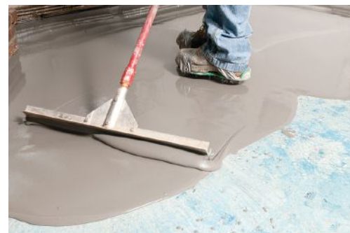
Cementitious, self-leveling underlayments are recommended to achieve flatness requirements.
