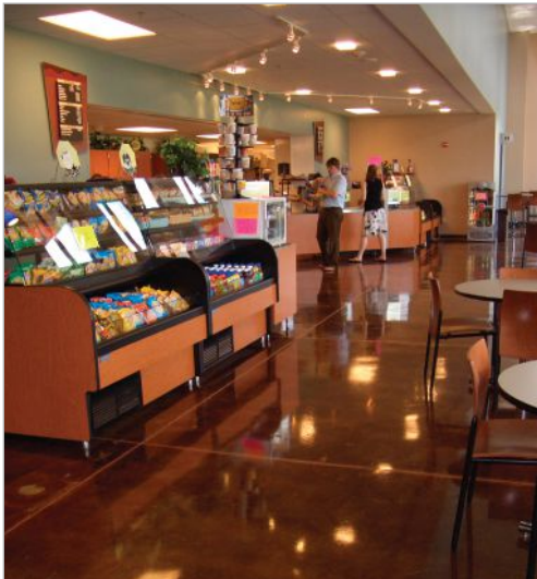
Interior joints on horizontal surfaces that see traffic such as this decorative stained concrete floor can be sealed to make cleaning easier.
