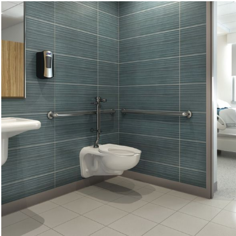
This healthcare bathroom includes a wall-mounted water closet and flushometer and a lavatory with a sensor-activated faucet. Note the grab bars and clearances around the fixtures.
