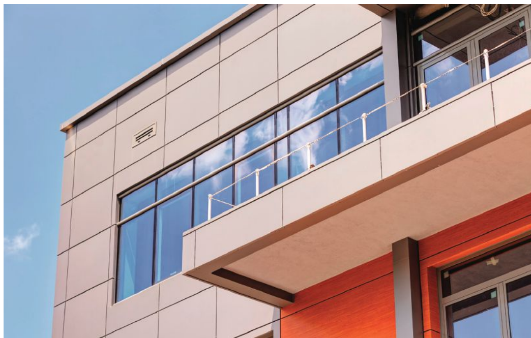
High performance joint sealants prevent fluids, like wind driven rain, and air from passing through a filled gap while staying adhered to a substrate that can move for environmental and structural reasons.
