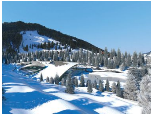
The Grandes Combes Courchevel blends with the snowy landscape to preserve the pristine vistas of the French Alps. Photo courtesy of Auer+Weber+Assoziierte GmbH.
