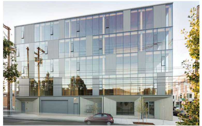
To mitigate solar gain, the main glazing appears on the north and west facades. Note the operational windows, allowing occupants to take advantage of Portland's mild climate and reducing energy expense on conditioned air.
