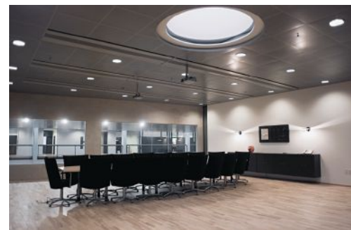
Chilled beams cool a room by circulating air through ceiling-mounted chilled water coils. Photo credit: Halton
