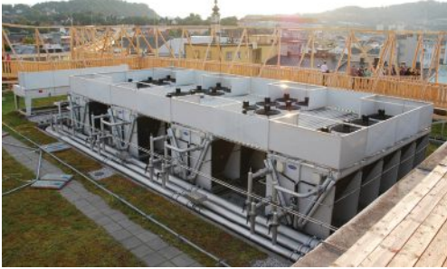
Air conditioners force refrigerants to continuously evaporate and condense in a closed system of coils.
