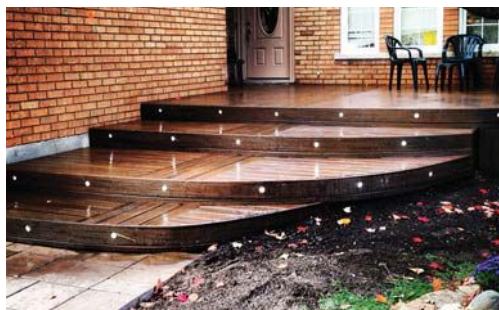
Not just another front porch. These unique steps are made with the latest in wood-alternative deck boards
