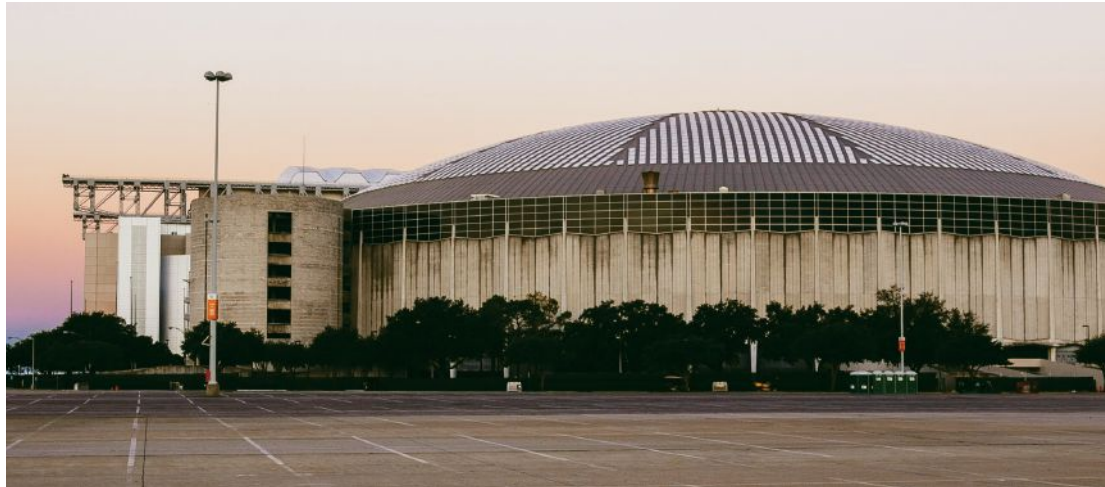
The Astrodome has a relatively modest silhouette, because the playing field inside was sunk 30 feet below grade.
