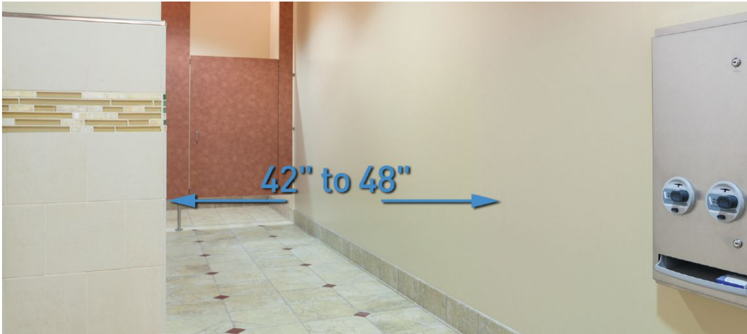
For large public restrooms passageways and access aisles are a minimum 42 inches to 48 inches to allow people using wheelchairs to maneuver around obstructions, such as sight-barriers, and to accommodate simultaneous in and out traffic. Credit: Bobrick Washroom Equipment, Inc.
