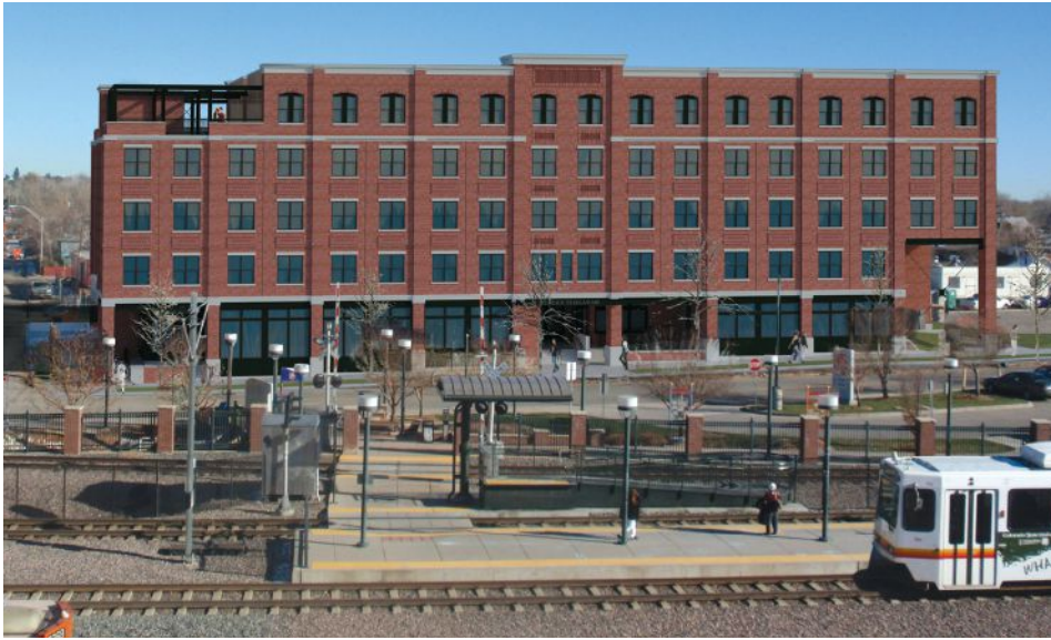
A light-rail station runs just in front of the Evans Station Lofts, an affordable housing project in south Denver designed from the ground up by Parikh Stevens Architects.
