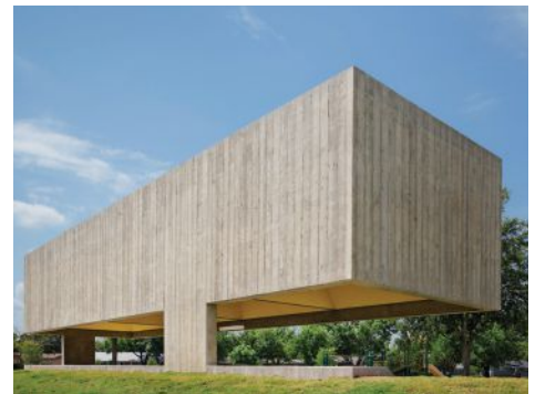
Webb Chapel Park Pavilion
