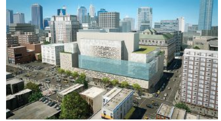
The Brooklyn Detention Center 1100 Architect/Ricki Greene
