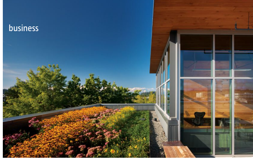
LOTT Clean Water Alliance Treatment Center • Olympia, Wash. • The Miller Hull Partnership • Class A reclaimed water that is treated and recycled at the plant facilitates the building's toilet-flushing and irrigation needs.
