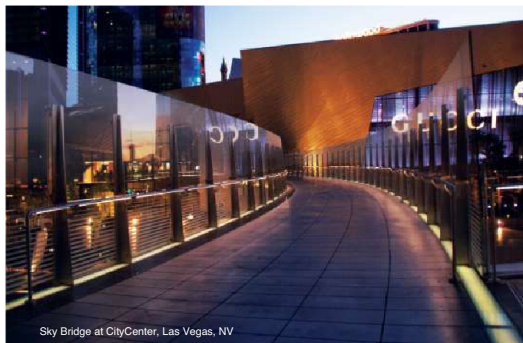
Sky Bridge at CityCenter, Las Vegas, NV
