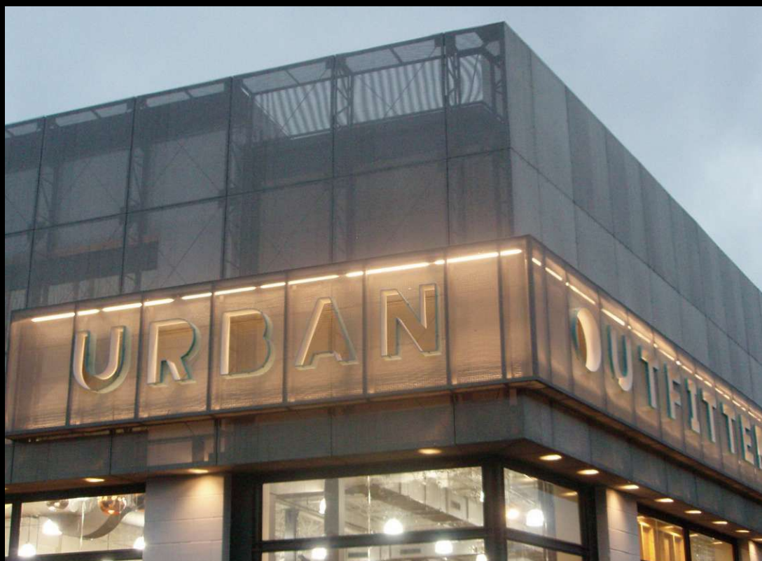
The trendy signage for the Atlanta Urban Outfitters store in Atlanta, GA, is made with McNICHOLS® Designer Wire Mesh.
