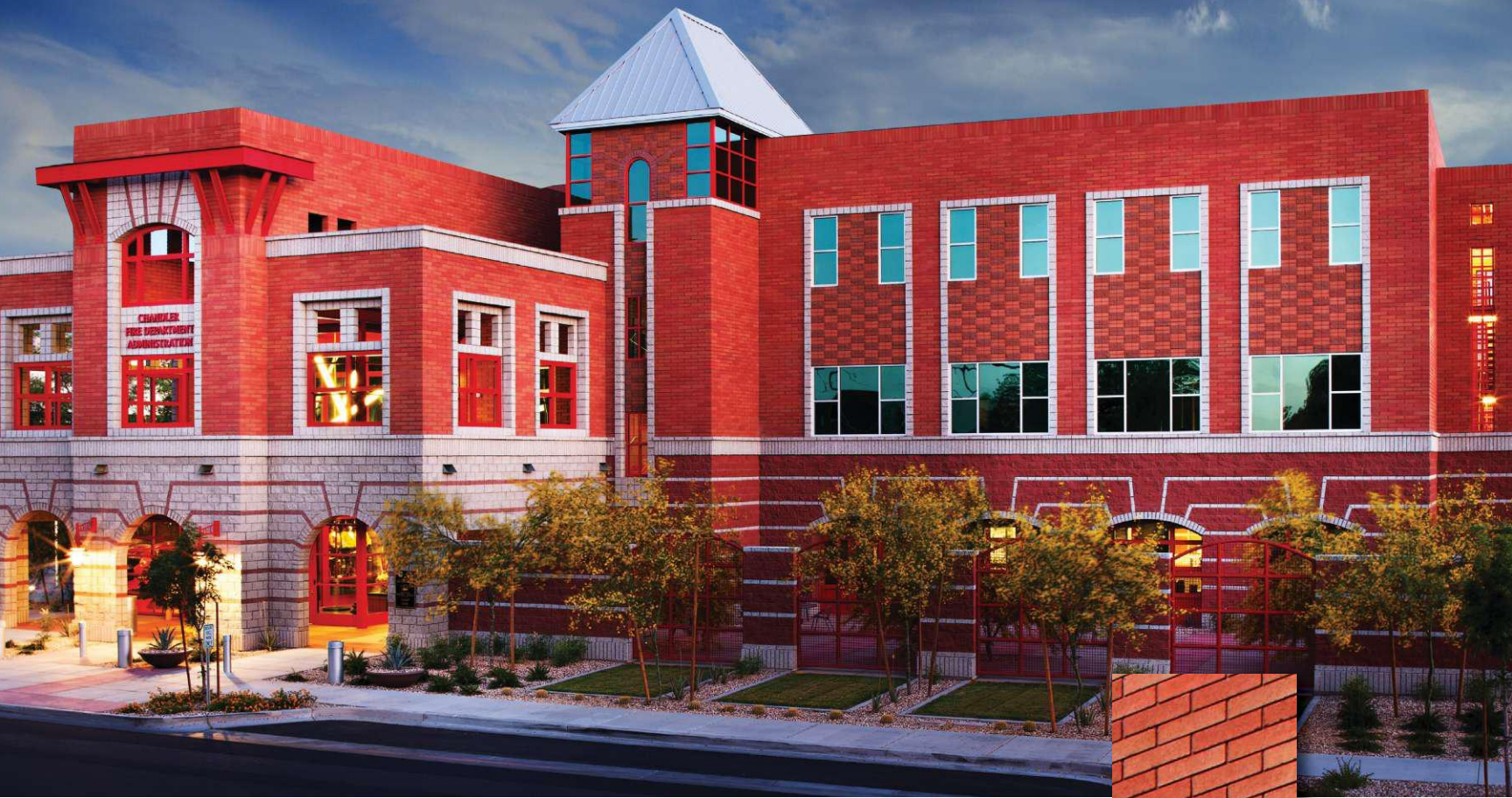
-Project: Chandler Fire Administration Building, Chandler, AZ.
