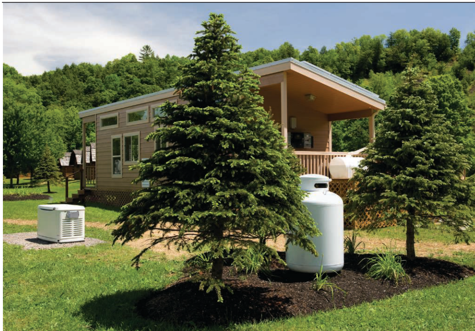
The propane generator used at the Herkimer lodge (small box to the left of tree) was specifically designed and built for off-grid applications. It is quieter than most generators and allows for 500 hours between servicing.
