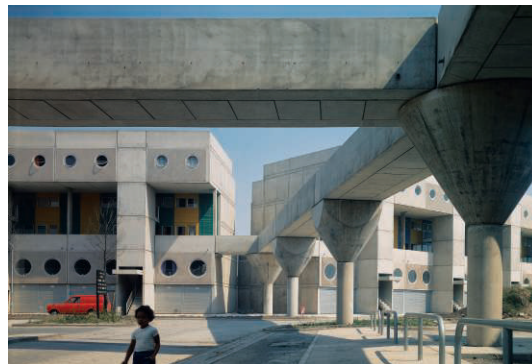
7. SOUTHGATE HOUSING, PHASES I AND IA, RUNCORN. TOP TO BOTTOM: AXONOMETRIC; PERSPECTIVE; ONE OF THE GEORGIAN-STYLE SQUARES; A COLONNADE AND RAISED WALKWAYS
