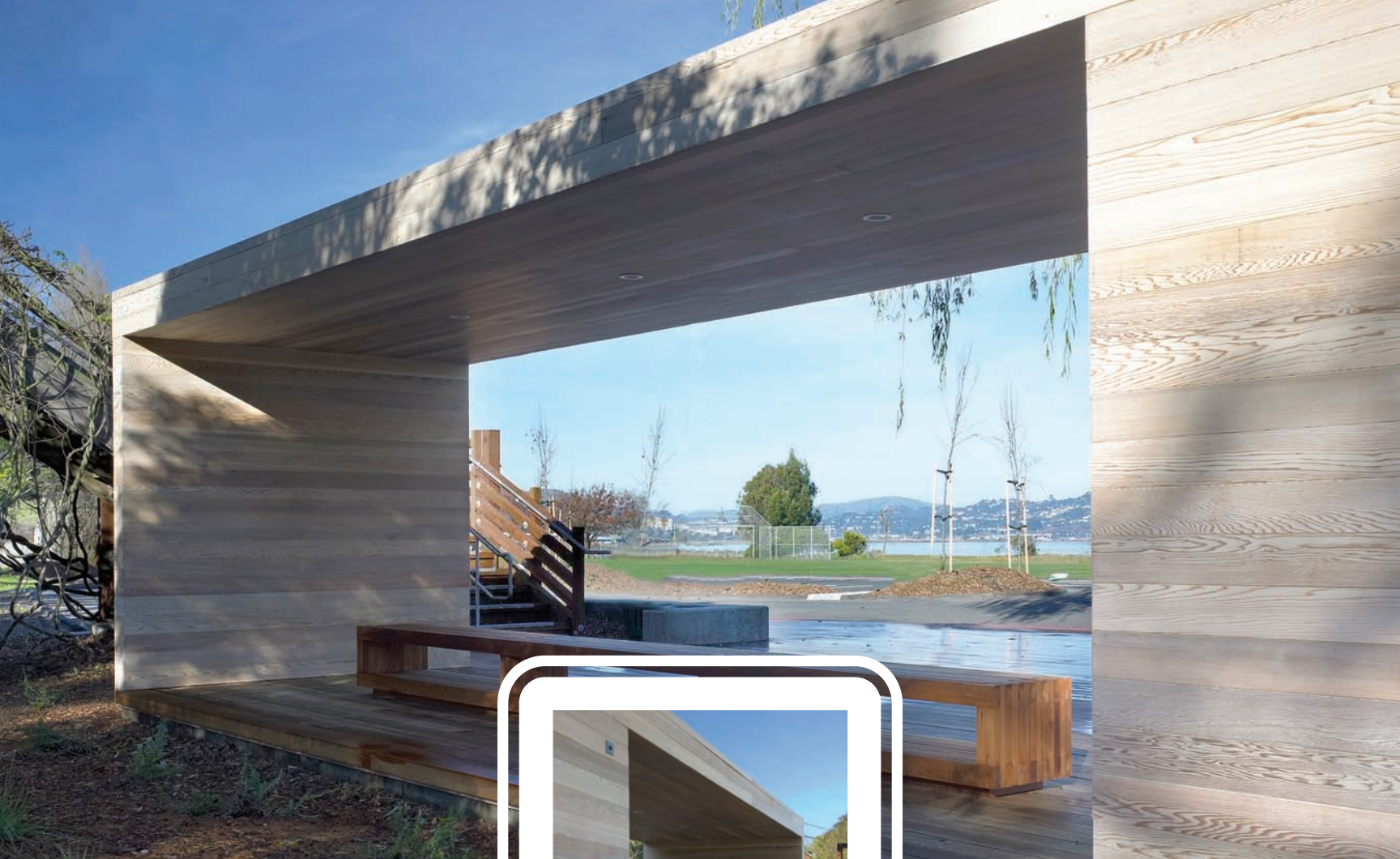
Marin County Day School Architect - Mark Cavagnero Associates Photo ©Tim Griffith
