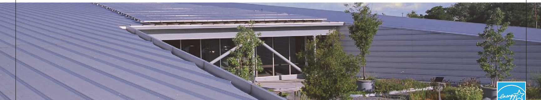
Bridges Center, Memphis, TN
