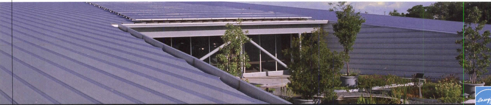
Bridges Center, Memphis, TN
