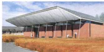
Among the new Greensburg buildings already completed is the 5.4.7 Arts Center (top), which opened in May 2008. City Hall (above) and a handful of other structures should be finished by the second anniversary of the storm.
