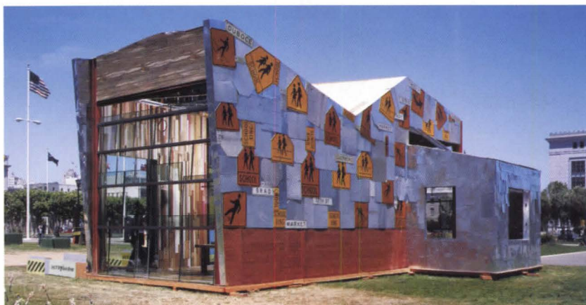
Public Architecture's recycled-metal-clad ScrapHouse was a demonstration project temporarily sited adjacent to San Francisco's City Hall.
