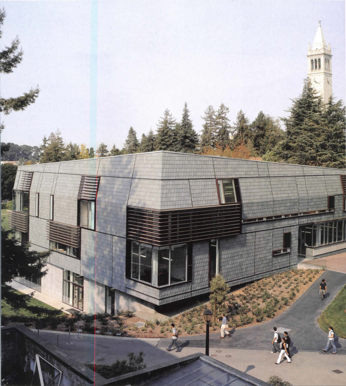
74 Mack Scogin Merrill Elam Architects' slate-shingle-clad design for the Jean Gray Hargrove Music Library at the University of California, Berkeley adds a fourth edge to the campus' arts quadrangle.
