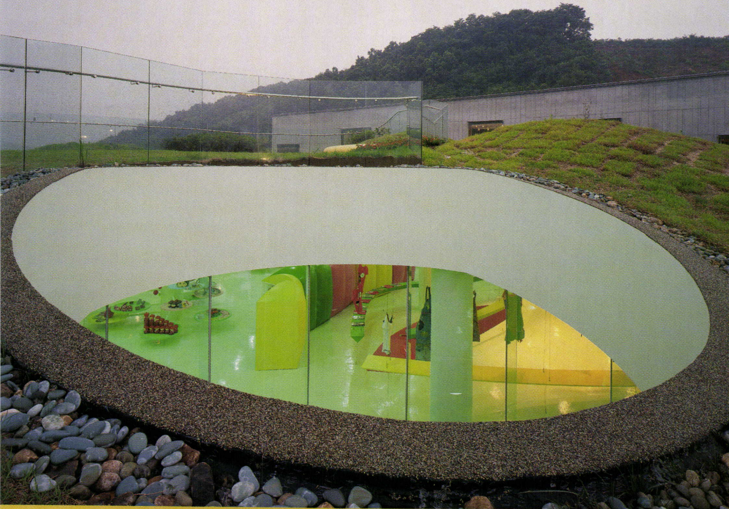
Bubbles, blisters, and tubes intersecting the main spaces offer shortcuts between levels and activities. Originally planned to contain a slide, a light shaft (above) instead offers visual connections between spaces.
