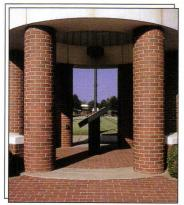
ral colors that resist ultraviolet radiation, which can cause fading in many artificially colored concrete pavers. Modular or 8-inch paving bricks are available with three edge detailssquare, chamfered, and lugged—in both mediumtraffic and vehicular-traffic grades, all of which are suitable for mortarless sand-set installations.
