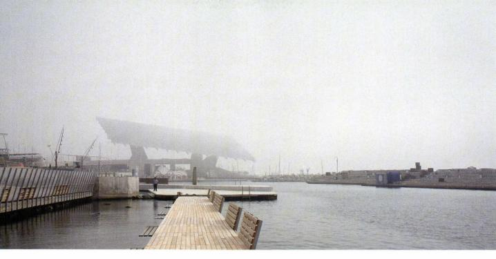
Adjacent to Galí's beachfront is the 113,000-square-foot solar collector (above and below) designed by Elías Torres and José Antonio Martínez Lapeña. Facing south at a 35-degree angle, its 3,700 photovoltaic cells can generate 1.3 megawatts of power.
