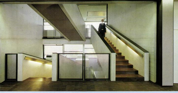
The architects offset two linear office wings in both plan and section, creating a split-level system of connections between floors. This vertical circulation becomes part of the open-plan workplace. The ramplike staircases have oak treads and handrails of folded stainless-steel plates with integral downlights.
