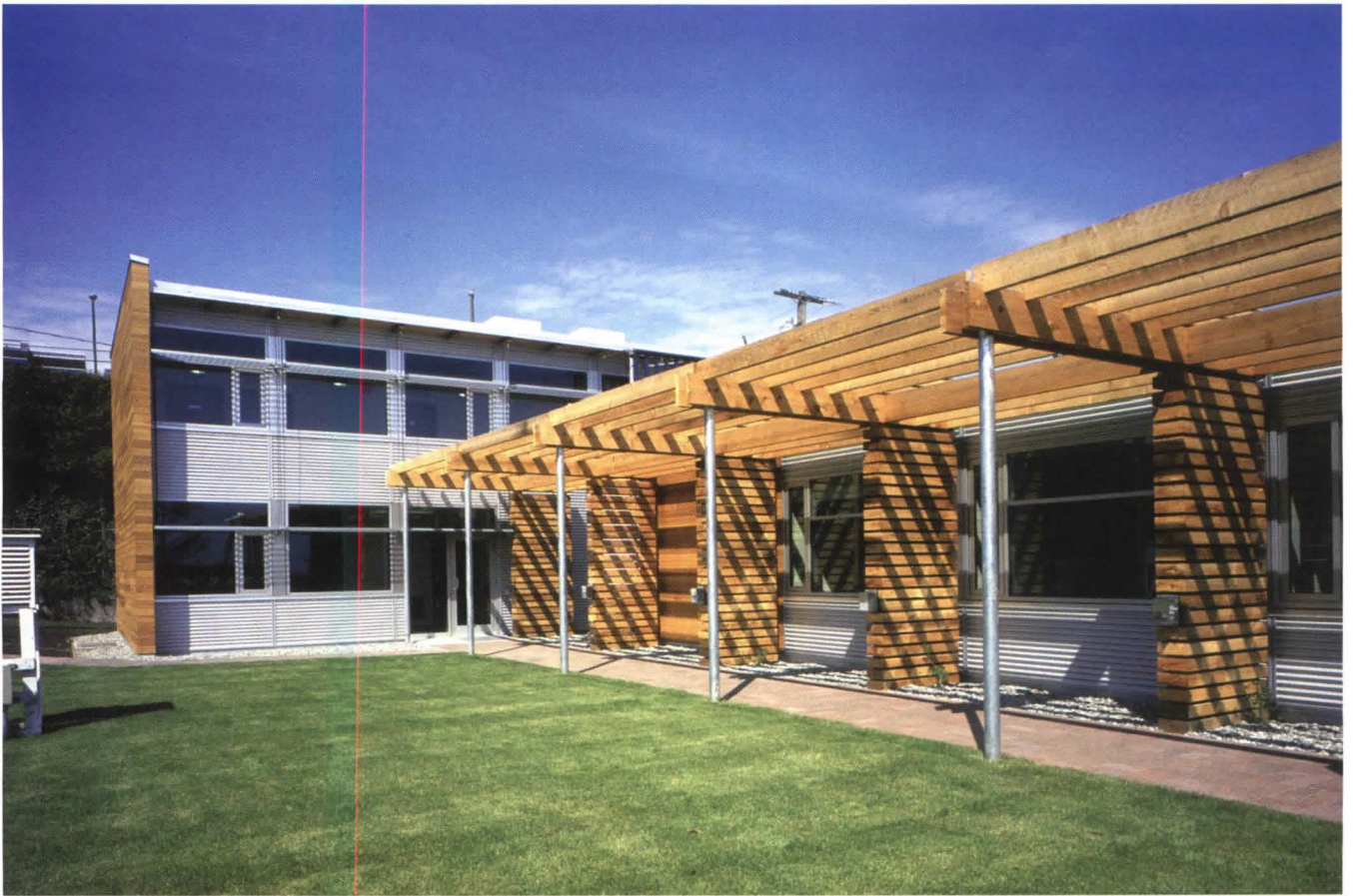
An east-facing trellis leads to the front door of the crew facilities. Since these photographs were taken, vines have been planted at the base of the wood walls of the trellis, and panels of photovoltaic cells have been added to its roof.
