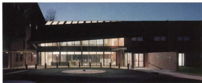
The 1885 St. Joseph's Academy for Girls once welcomed visitors through a stately streetfront entrance (top). Now transformed for senior living, the Clare Estate's main entrance (above) is situated in the complex's courtyard, leading into a new wing.
