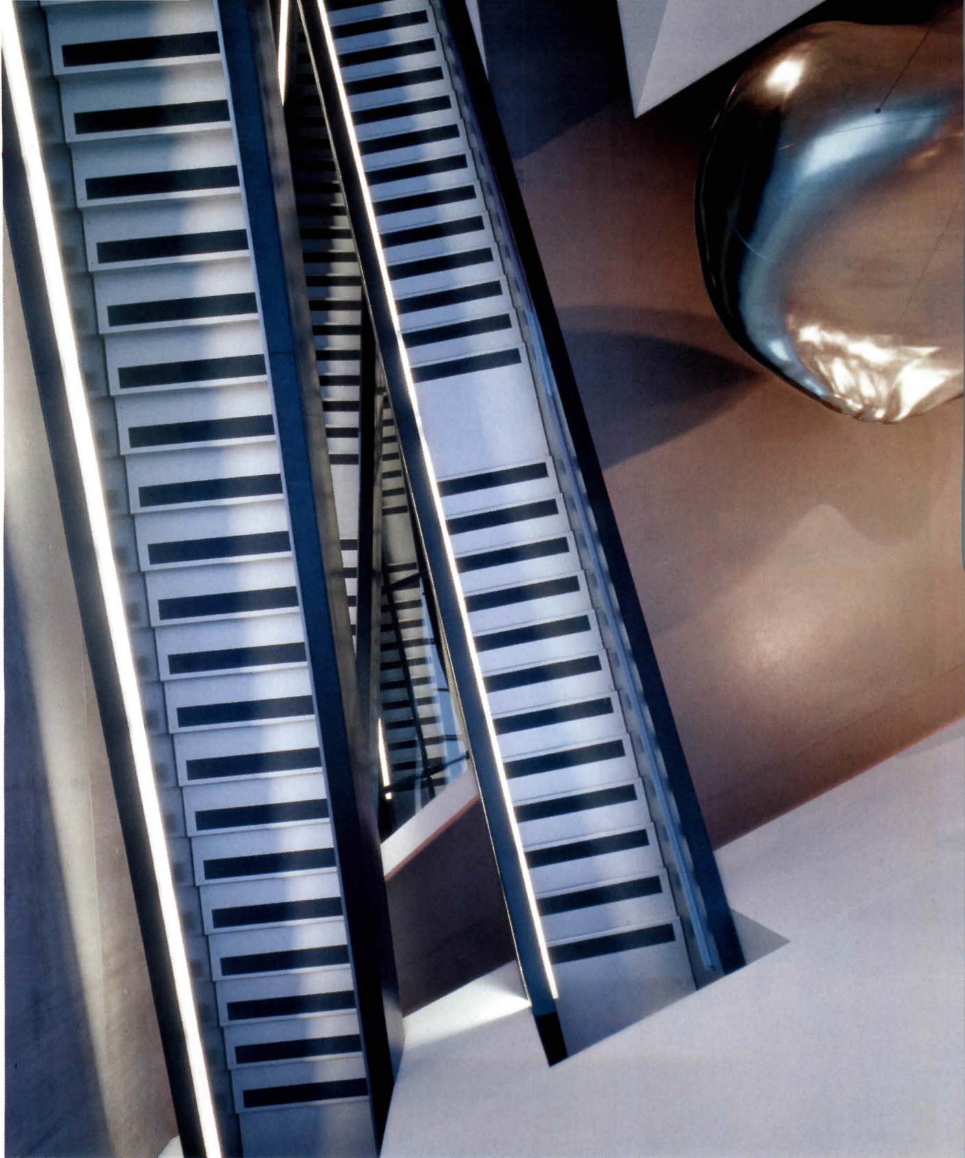
Ramped steps, with intentionally low risers and deep treads, speed movement up and down the dizzying circulation core. Each ramp is of equal length; only their ends are unique, tailoring them to individual portal conditions through which they seem to bust their way at various angles.
