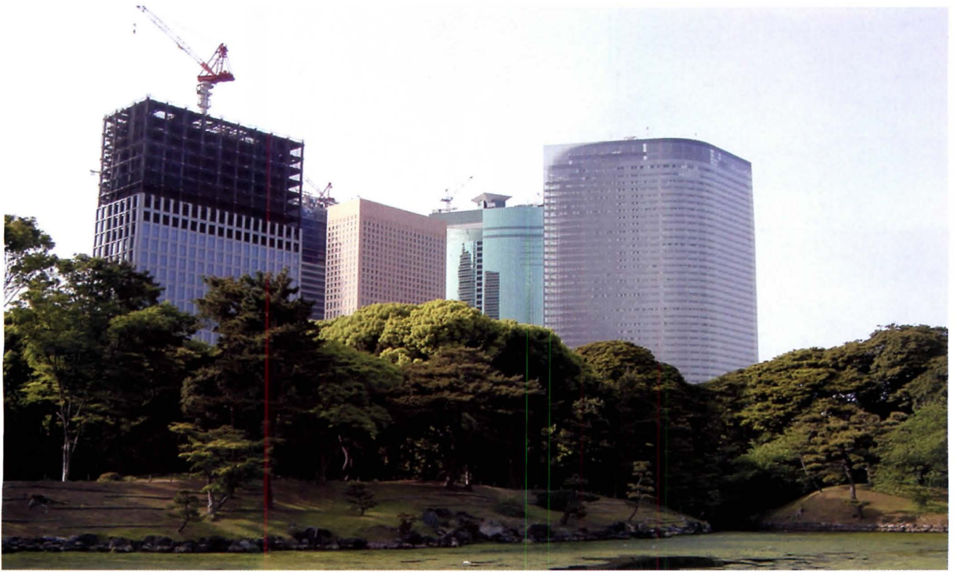
Nouvel's bowed plan was intended to help reduce the building's impact on a nearby park, while simultaneously providing as many employees as possible with a view of the green space, one of few in Tokyo. Dentsu is part of a growing office development called Shiodome.
