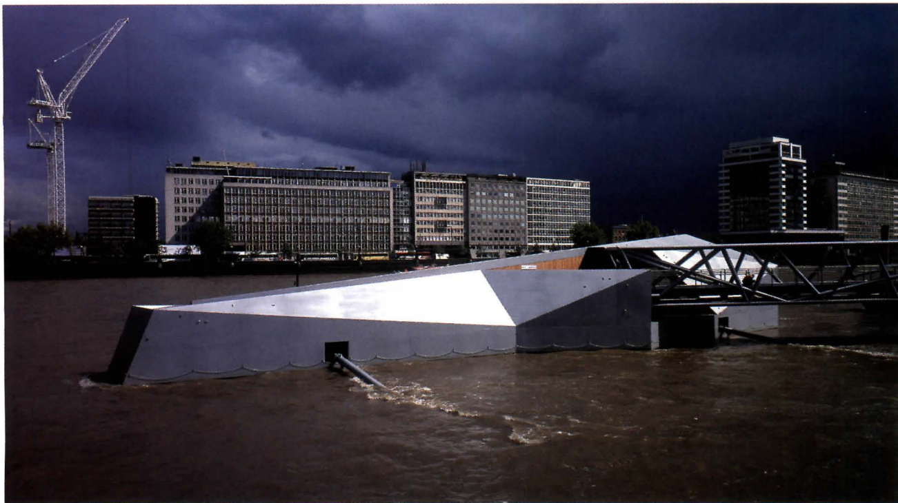
Traditional pontoon construction involves welding steel plates together to form a floating box, but at the Millbank Millennium Pier a continuous surface of steel plates integrates ramps, steps, and pontoon shelter (above). An extra long brow (facing page), fixed-gradient ramps, and a stair on the pontoon maintain a one-in-twelve gradient for disabled access throughout the Thames's 20-foot tidal range.
