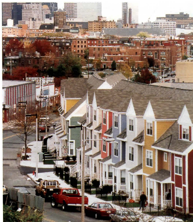
At the Orchard Gardens development in Boston's Roxbury section, wood-frame townhouses built through the Hope VI program nod to the vernacular of the neighborhood.
