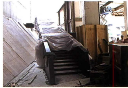
Each steel ramp was fabricated off site by a manufacturer of roller coasters and lowered into place by a crane after the main structure was complete (left). While the galleries are sealed off from natural light, with the exception of those in the "Unmuseum," the circulation core reconnects visitors to the city through east-facing glazed walls; glazed ceilings and other devices create four individually controlled climate zones (right).
