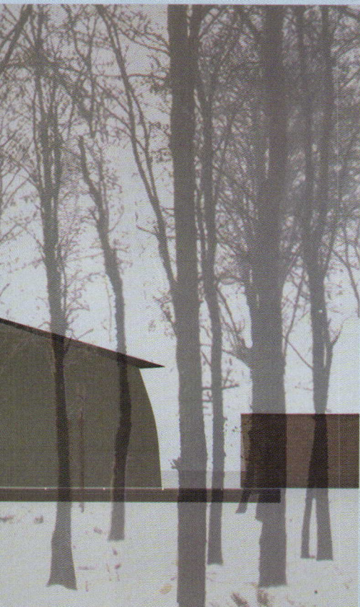
East façade and viewing courtyard through a stand of trees
