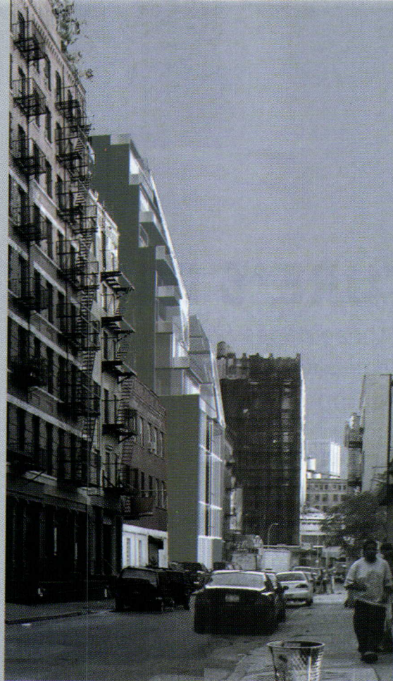
View from north along Renwick Street
