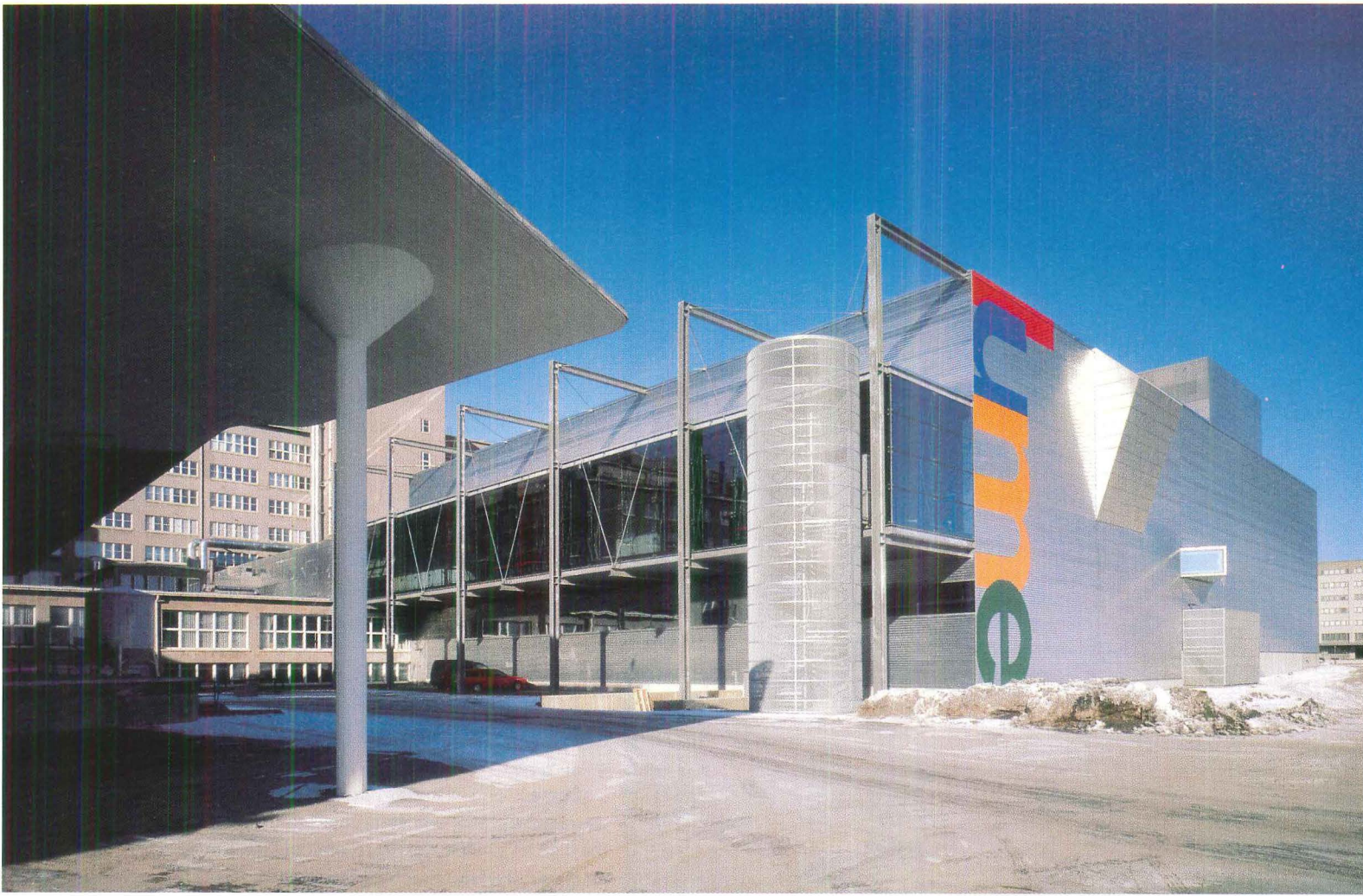
A glazed "bridge," fronted by a metal mesh-clad stair tower, runs the length of the media center's south face. The bridge is supported by I-beams cantilevered from the main addition as well as from a subsidiary system of cables.
