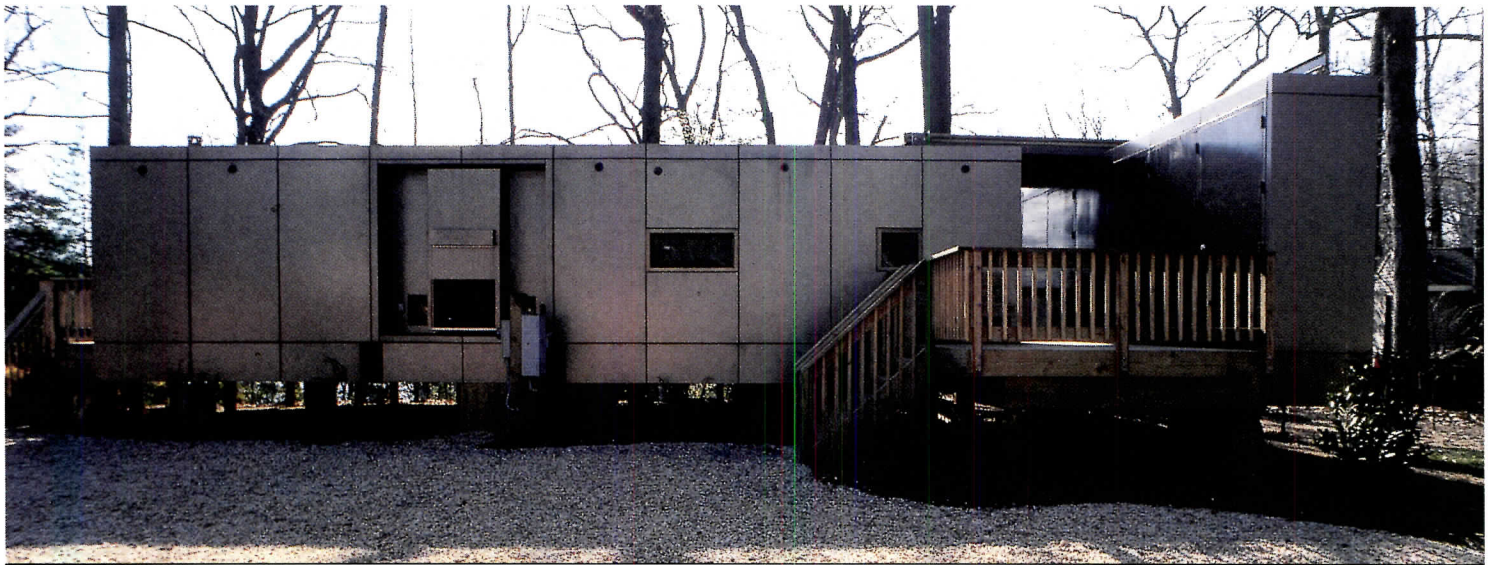
PERMANENT SETTING Catholic University's Nomadic Transit Module (NTM) is now situated on a wooded site along the Severn River, near Annapolis, Maryland, where it was shipped on the back of a flatbed truck, like a mobile home. The enclosed north elevation (above) conceals the NTM's services; a small, freestanding "battery barn" (at right) was designed to house energy-generating equipment. (The current owner elected to hook up the house to the local grid instead, and is currently using the shed for storage.)
