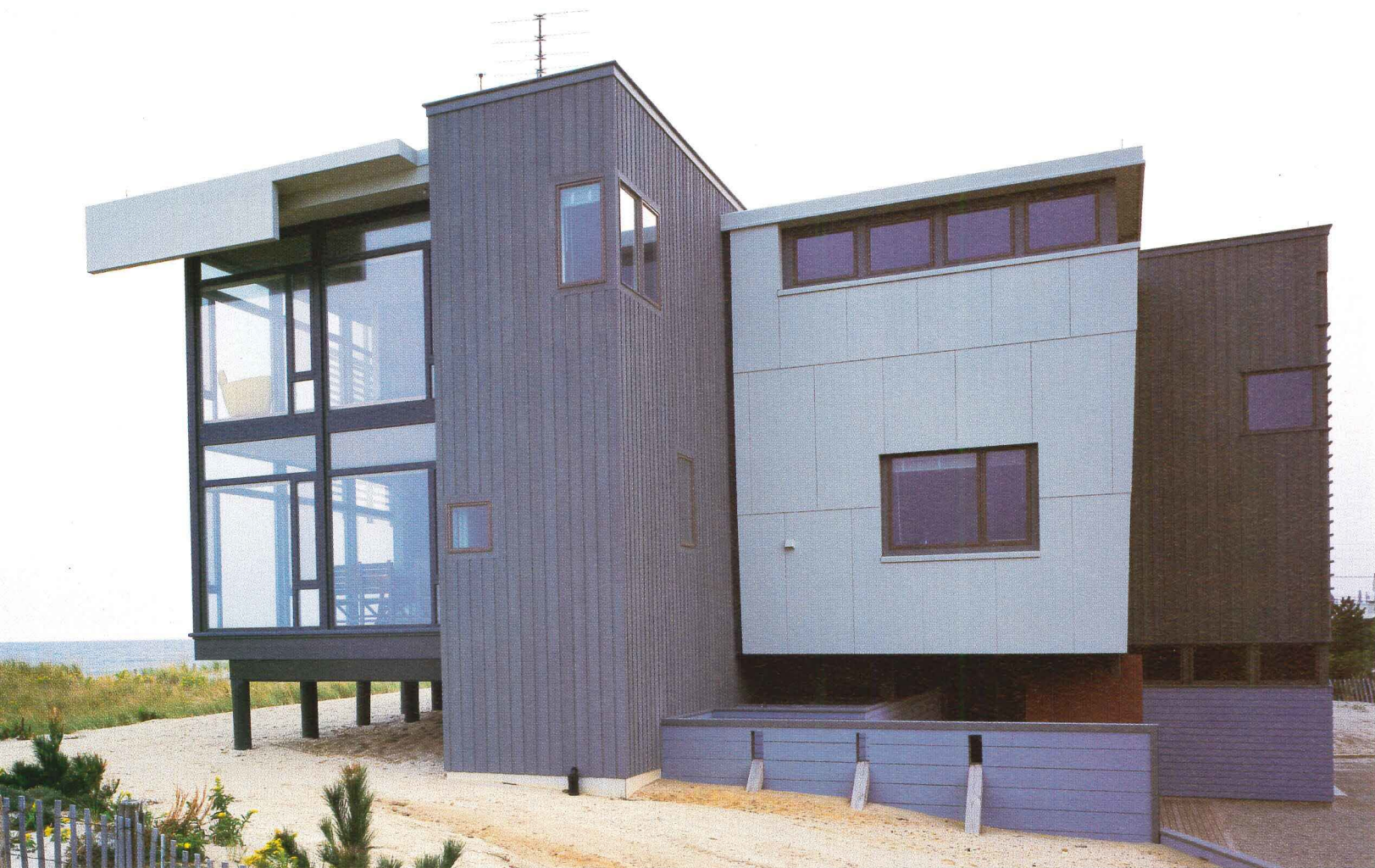
Fiber-reinforced cement panel-clad kitchen and stained cedar-clad bedroom block (top left) step back from driveway at northwest corner. Glassy east facade of living room (top right), screened by grid of wooden louvers, faces beach. Stair tower on north facade (above) mediates between glazed living room and angular box containing kitchen.
