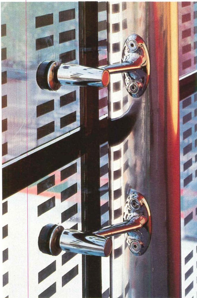
At Palais de Beaux-Arts extension in Lille, France, each facade panel (above) attaches to elliptical stainless steel tubes by four cast stainless-steel brackets, which support articulated bolts within glass unit. Layered glazing of north facade (facing page) reflects an impressionistic image of the 19th-century museum's south facade.
