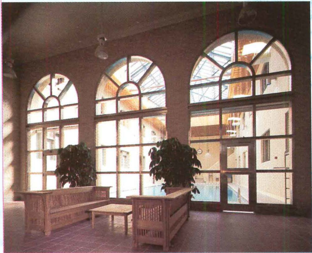
Glazing arched, 18-foot-tall windows between entrance hall and natatorium reopened lines of sight between central portal and pool.
