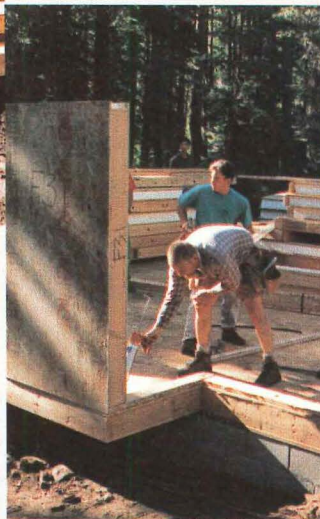
Workers prepare wall-to-floor connections with sealant and adhesives.
