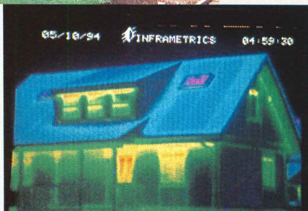
Infrared photograph (above) of SIP demonstration house in Springfield, Oregon (top), reveals high energy performance with low incidence of thermal breaching (indicated in yellow). Intended as production housing prototype, house was sponsored by Energy-Efficient Industrialized Housing Research Program of the U.S. Department of Energy and built by University of Oregon's Energy Studies and Building Laboratory and University of Central Florida's Solar Energy Center.
