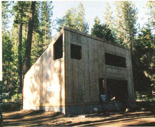
At end of day, shell of Wright house is complete.
