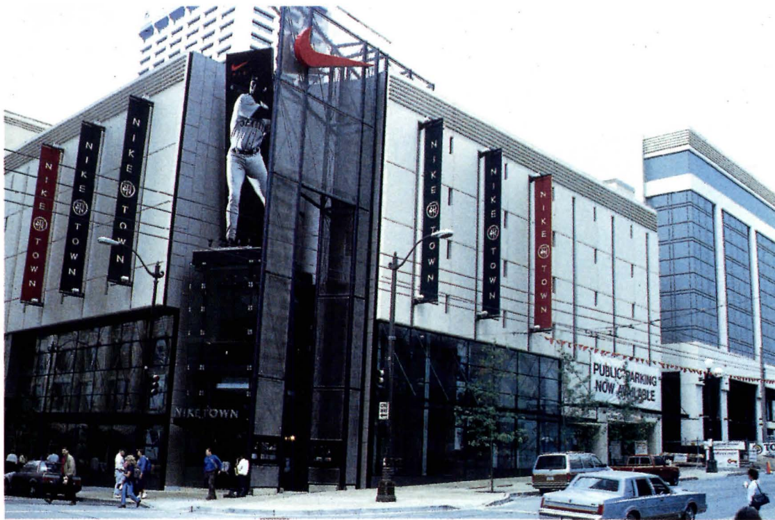
STYLELESS IN SEATTLE: Bland facades and strip mall detailing squander important urban site.
