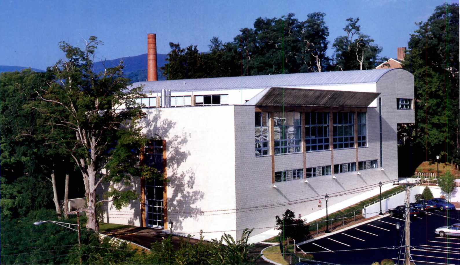
W.L.S. Spencer Studio Art Building Williams College Williamstown, Massachusetts Carlos Jimenez Studio, Architect
