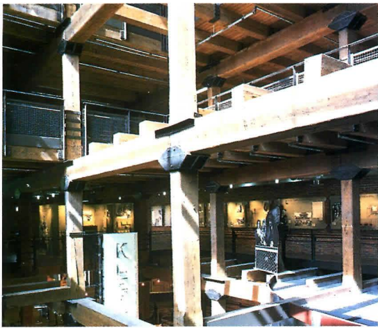
TIMBER FRAME: Opened to create seven-story atrium.
