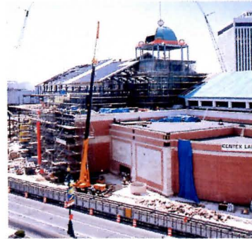
CASINO: Construction stalled.
