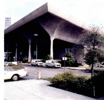
RIVERGATE: Now demolished.
