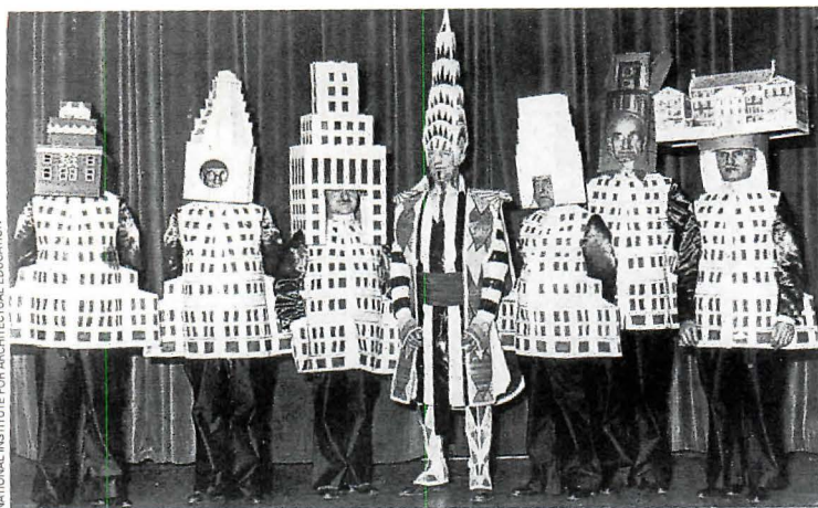
ARCHITECTS AS BUILDINGS: 1931 Beaux-Arts Ball, including Van Alen (center).
