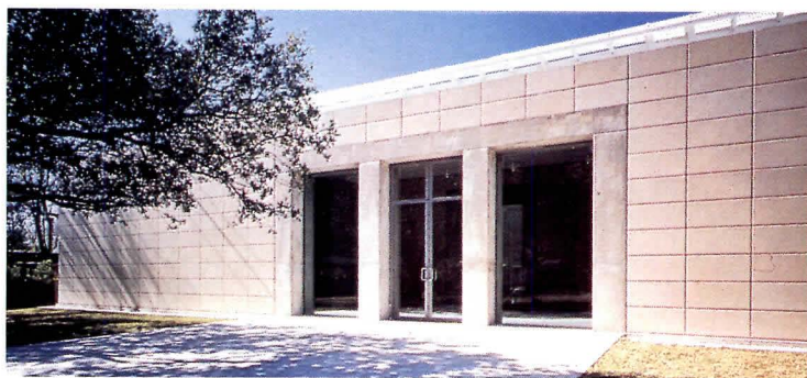
GALLERY: Precast concrete surrounds entrance framed in poured concrete.
