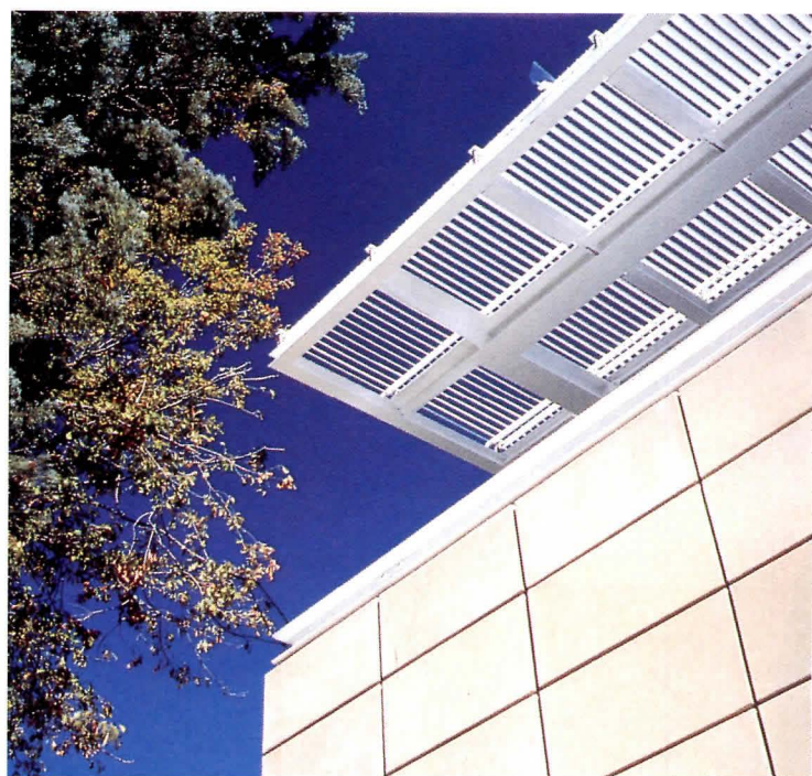
ROOF DETAIL: Steel grille above skylights in roof screens daylight.
