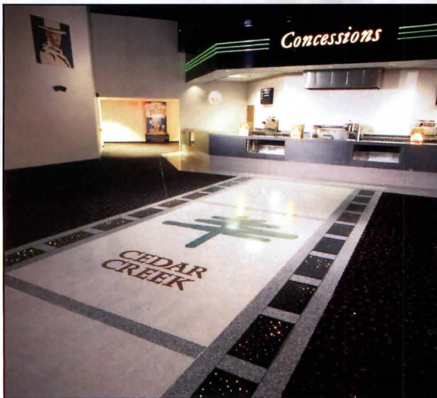
Terrazzo Tile Using Water-Jet Cutting In Combination With Embedded Fiber- Optics, Giving Intermittant Sparkling Light Transferred Through the Terrazzo Floor.
