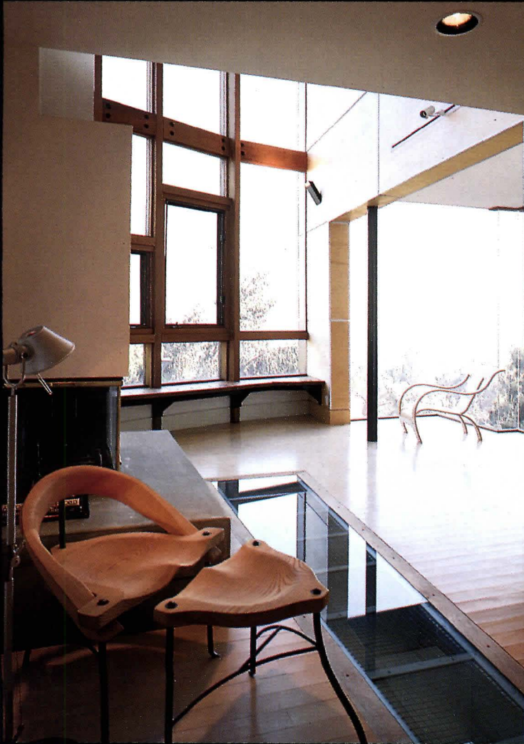
DETAIL OF GLAZED FLOOR OVER POOL
