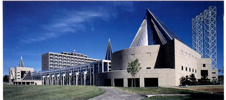
COLLAGE: Glass cones and pyramids top entrance pavilion (left) and council chamber.
