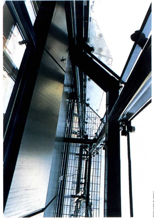
VENTILATED CAVITY: Incorporates catwalks.
