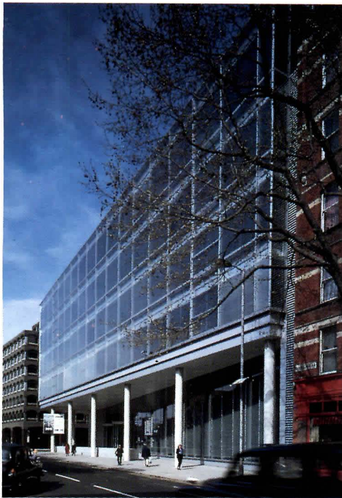
WEST FAÇADE: Compartmentalized cladding.
