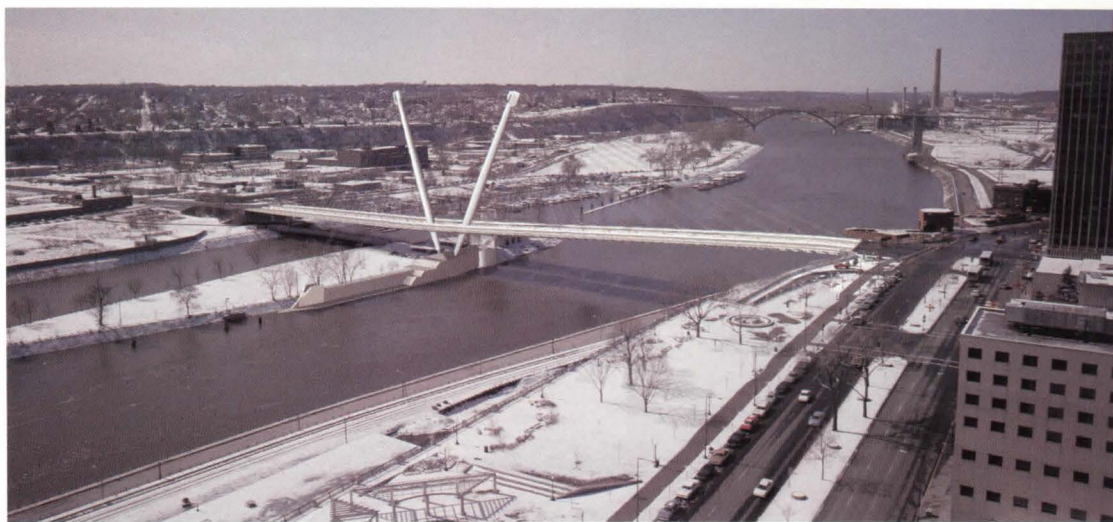
CABLE-STAYED BRIDGE: Proposed V-shaped mast incorporates island beneath bridge into pedestrian promenade across river.
