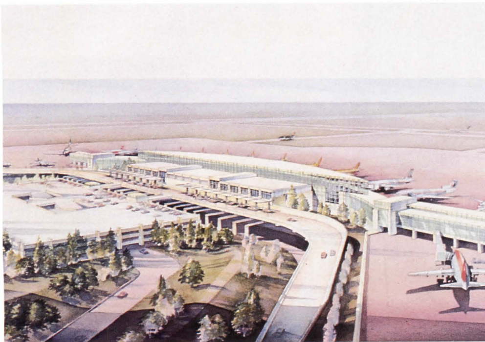
AUSTIN TERMINAL: Crescent form of 24-gate facility is designed to expand to 32 gates despite limited area of site.
