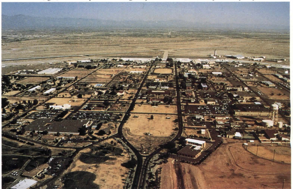
WILLIAMS AFB: View to east shows axis of training ground, which abuts airfield (background).
