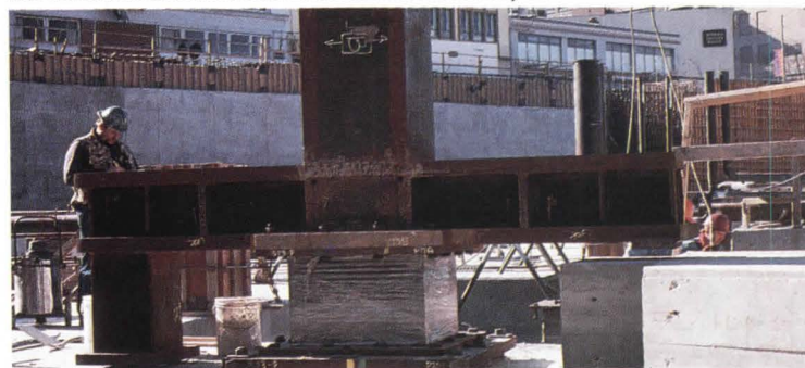
BASE ISOLATORS: Seismic devices cut $6.5 million in reinforcing costs.
