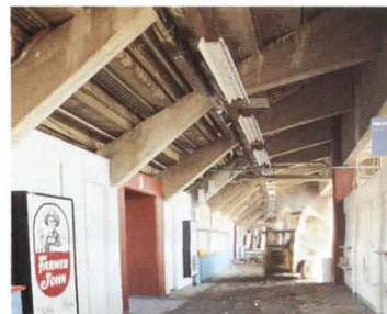
TUNNELS: Shored beams and columns.
