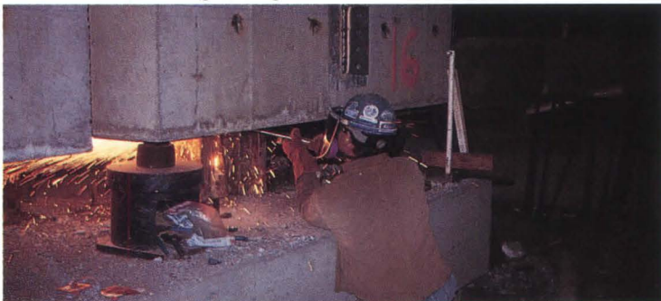
ON-SITE RETROFITTING: Existing column is jacked up and cut.
