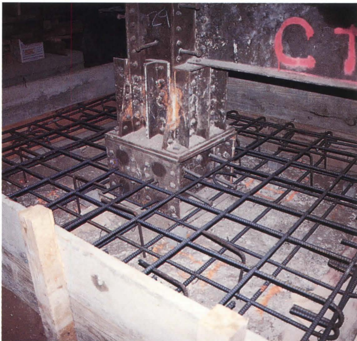
FOOTING: Column is strengthened prior to base isolator installation.
