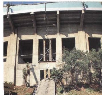
EXTERIOR: Weakened areas reinforced.
