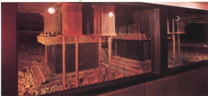
LEAD-RUBBER ISOLATOR: Inserted under column.
