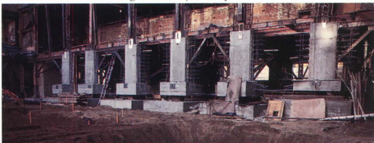
ISOLATOR INSTALLATION: Friction-pendulum dishes rest on bearing point.
