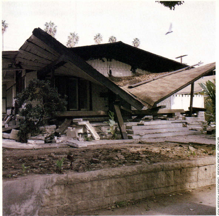
COLLAPSED PORCHES: Historic 1920s wood-framed bungalows severely damaged.
