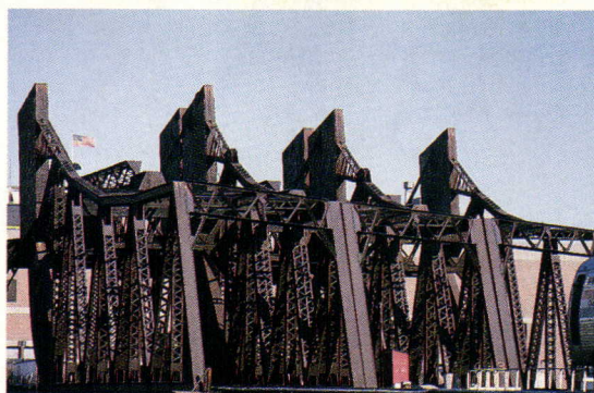
STEEL TRUSSES: Support active rail lines.
