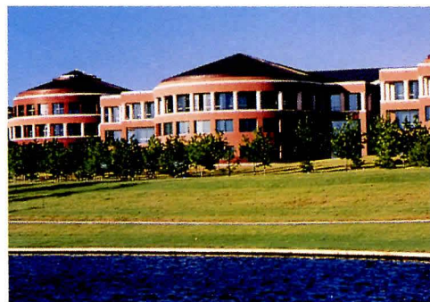
PENNEY HQ: One of the largest brine-cooled structures.
