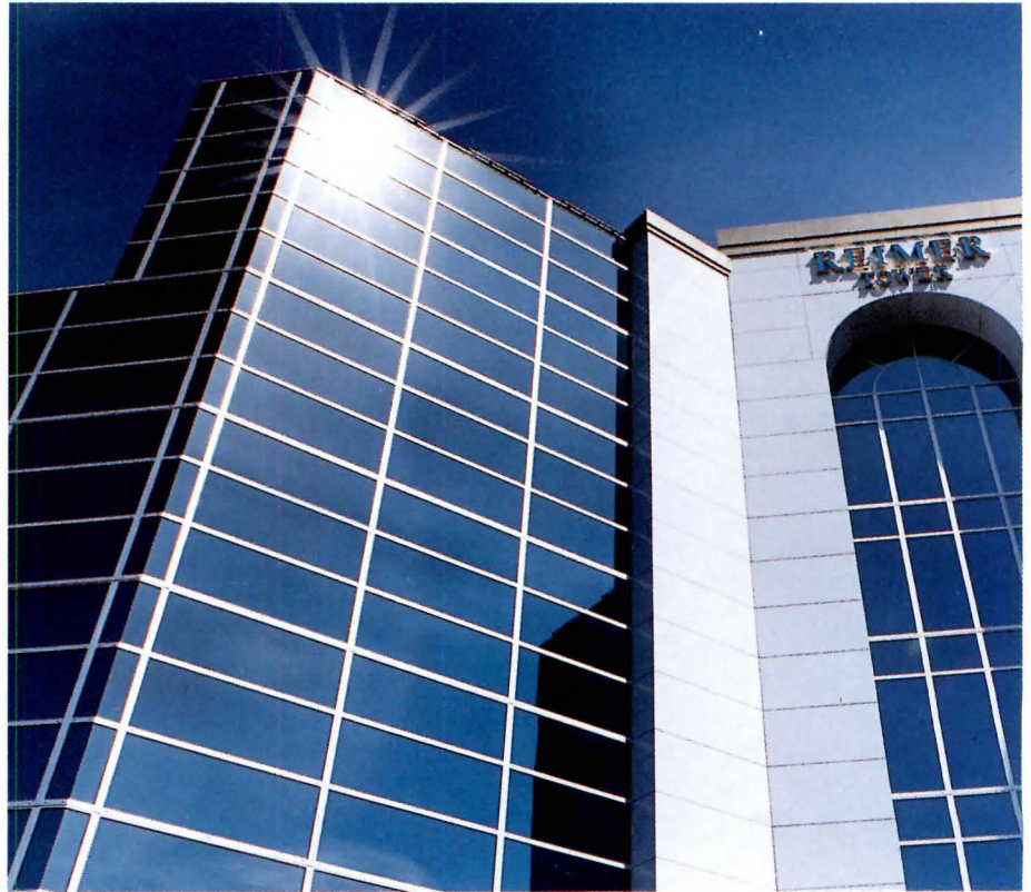
The Reimer Tower in Burlington, Ontario features VISIONWALL curtain wall without any form of perimeter heating.
