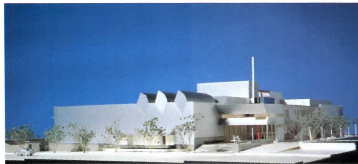
YUERBA BUENA GARDENS VISUAL ARTS CENTER: Under construction in San Francisco.
