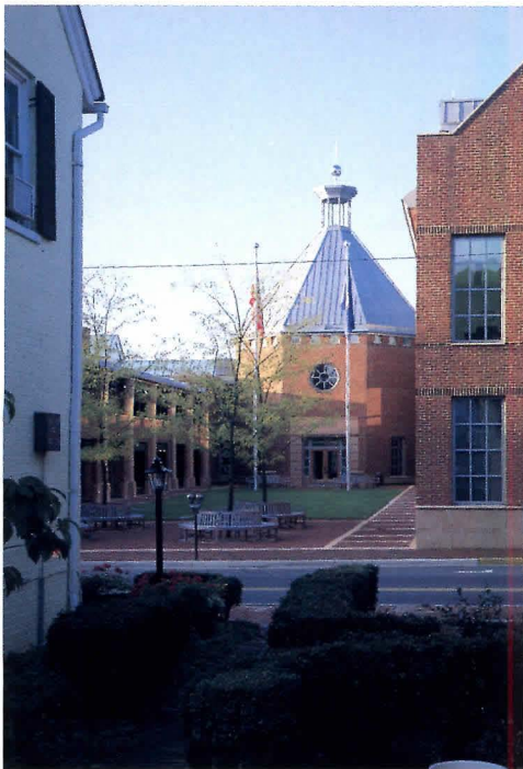
ABOVE: Architect Hanno Weber's plan for the government complex yielded many dividends, including a neatly defined urban plaza facing busy Market Street. BELOW: The center's three-story office building re-creates the urban edge along Wirt Street.
