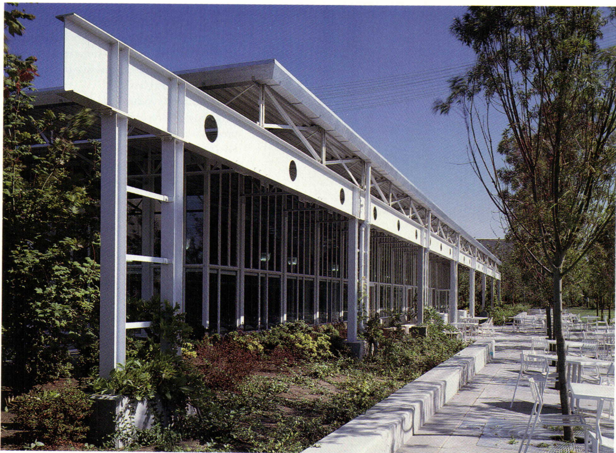
Glassy facade of Boeing Cafeteria 9-12 with steel sun screen of I-beams and columns (left and facing page, top) encloses 3,900-square-foot dining room (facing page, center). Section (facing page, bottom) reveals entry, servery, and dining room. Steel beams support entrance canopy (top left).
