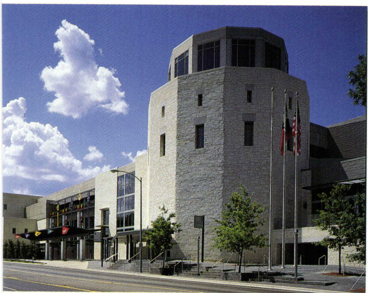
Austin Convention Center's energy savings are achieved through a variety of strategies. Deep porches and aluminum fins on west facade (facing page, top and bottom left) block sun during hottest hours, then admit late-afternoon light. South facade (left and facing page, bottom right) includes deep entrance overhang, screening all but indirect light.
