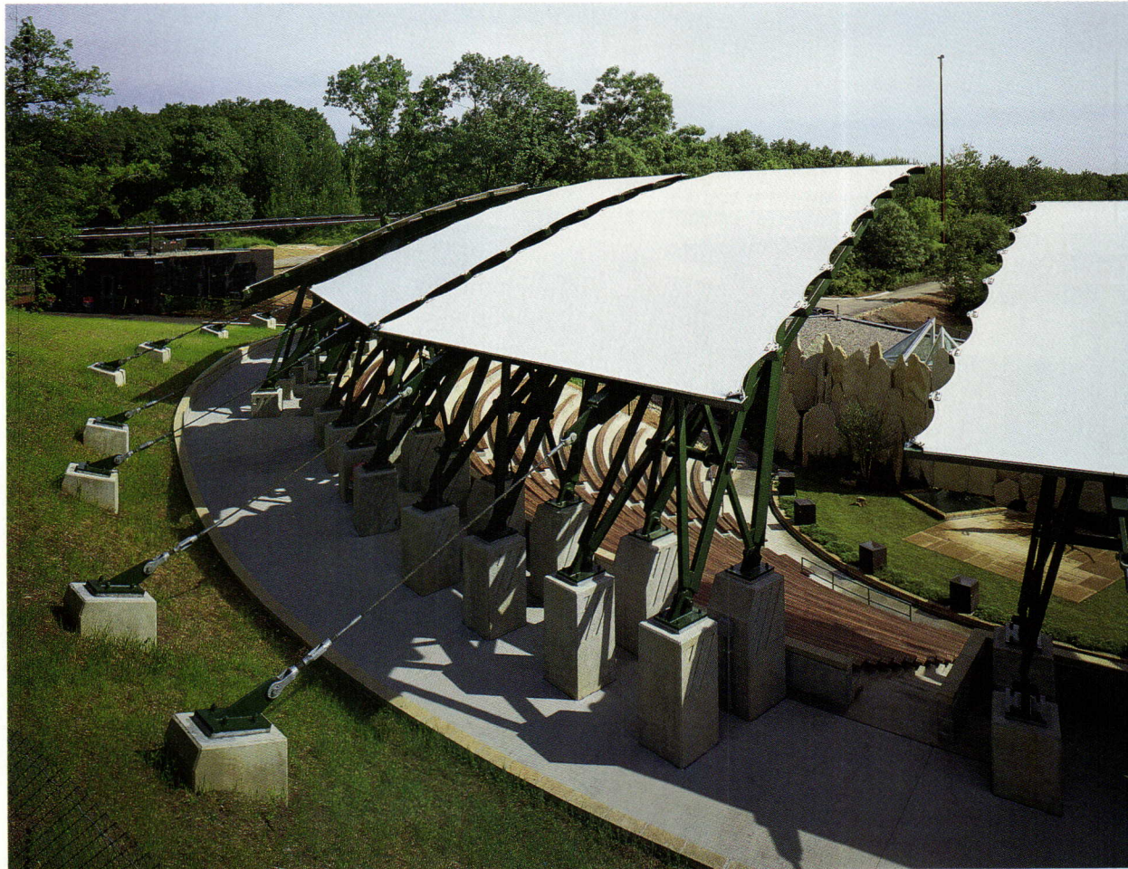
Nestled into a knoll along a lake (top), the curving amphitheater wraps a grassy stage (facing page, bottom and site plan). Three pairs of steel canopies are set on concrete bases (right) to compensate for the natural slope of the land (facing page, section).
