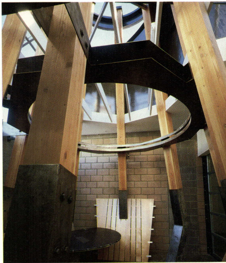
Gary Group Culver City, California Eric Owen Moss Architects
