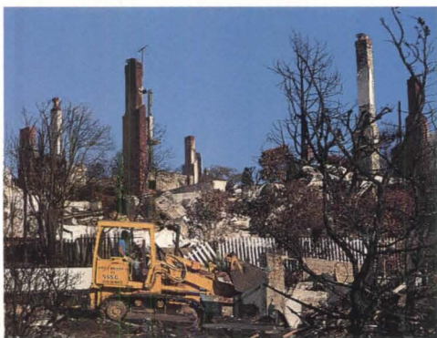
The fire scorched steep hillsides leaving only concrete and masonry foundations of many houses (top). Swirling winds spread the 1,800-acre fire through dry vegetation close to structures (second from top). The blaze was additionally fueled by unsafe building components including eaves and vents, decks, and porches. Shattered windows allowed fire to sweep inside houses, leaving only a shell (third from top) or chimneys (above).
