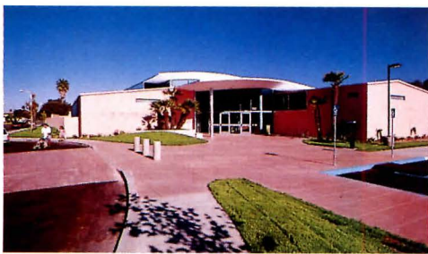
Ray D. Prueter Library Port Hueneme, California Scott Ellinwood & Associates, Architects
