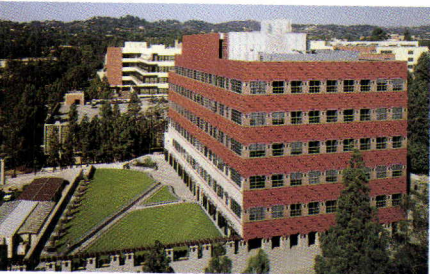
6 MACDONALD RESEARCH LABORATORIES FRANCESCO CENTURI, SCOTT BROWN AND ASSOCIATES AND PAYETTE ASSOCIATES, ARCHITECTS
