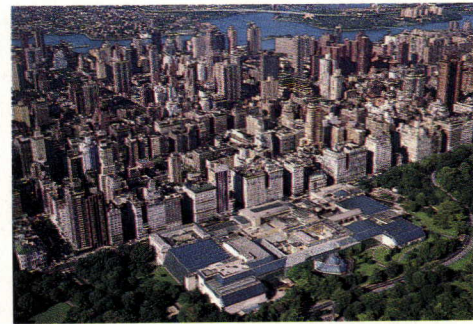
METROPOLITAN MUSEUM OF ART, NEW YORK CITY ARCHITECT FOR EXPANSION AND RENOVATION: KEVIN ROCHE JOHN DINKELOO & ASSOCIATES
